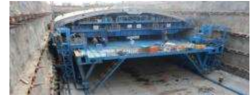
urban underground structure
