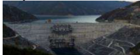
concrete arch dam
